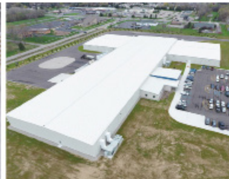
Fernco will continue to see the highest levels of quality and customer service.
